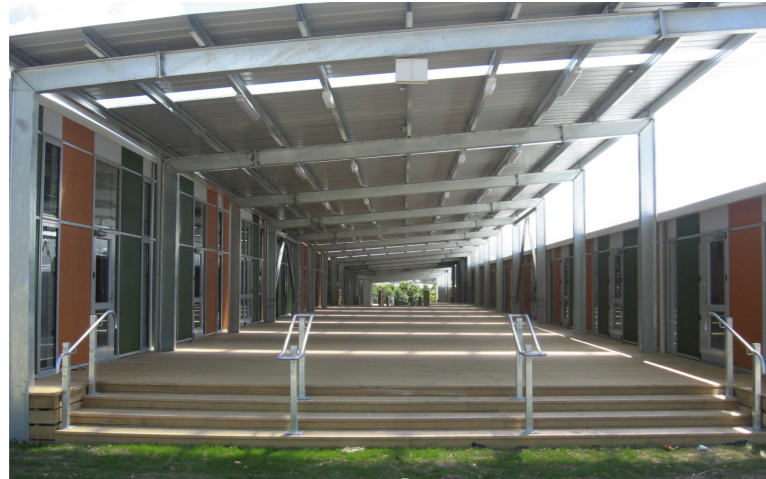
Albany Senior High Temporary School, Auckland / Jasmx
