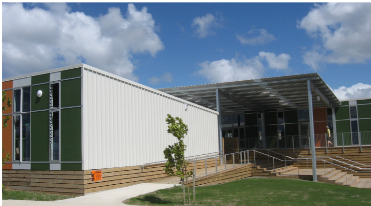
Albany Senior High Temporary School, Auckland / Jasmx
